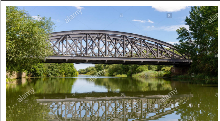
Windsor Railway Bridge (Brunel 1848) - 62 m
