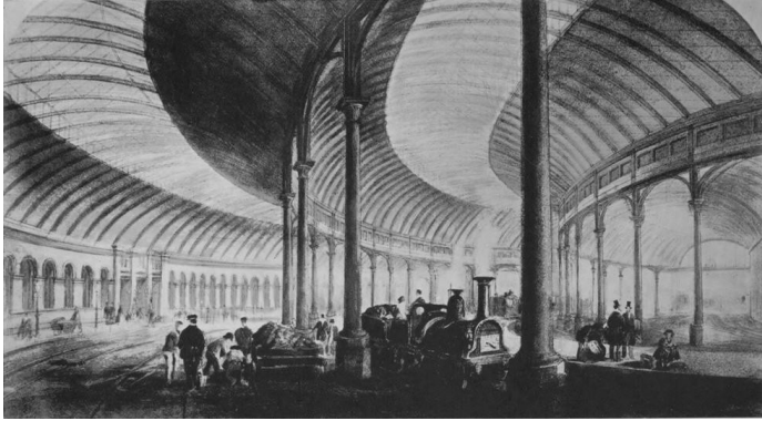
Newcastle Central station (1850)
