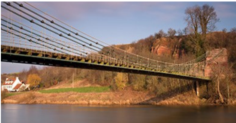
The Union Bridge over the Tweed (Brown 1820) – 137 m
