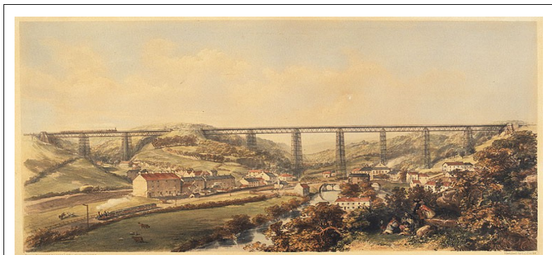
The Crumlin Viaduct (Kennard 1855) – 3+7×46 m
