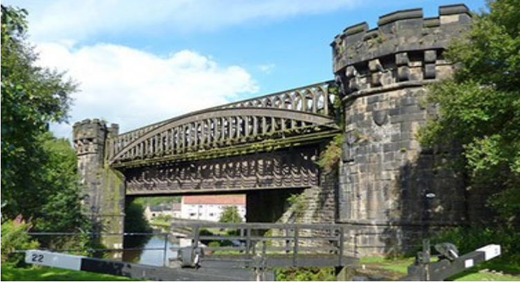
Gauxholme Viaduct (G. Stephenson 1840)
