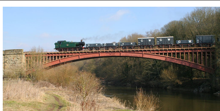
Victoria Bridge (Fowler 1864) – 61 m
