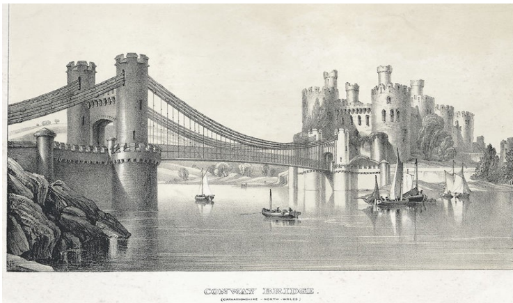
The Conway Suspension Bridge (Telford 1822) – 100 m
