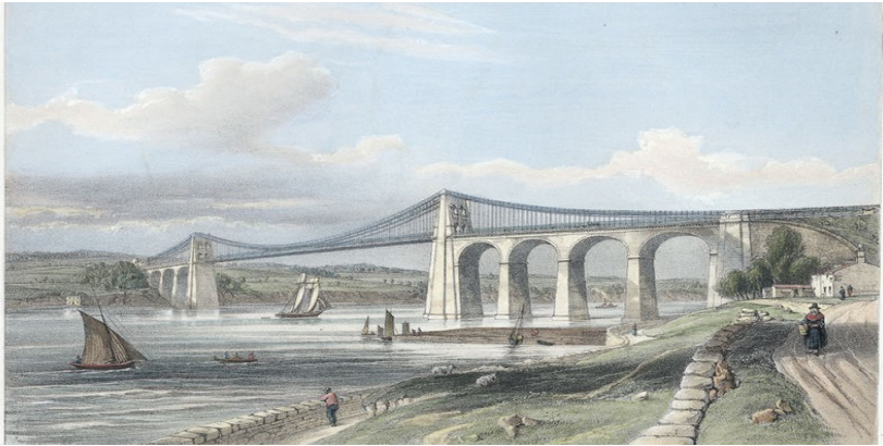
The Menai Straits Suspension Bridge (Telford 1826) – 175 m
