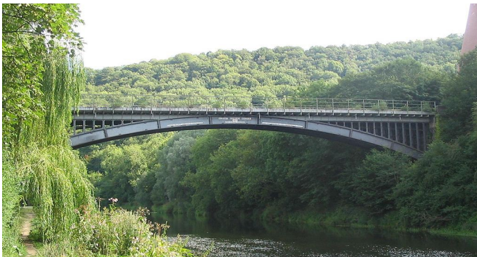
Albert Edward Bridge (Fowler 1864) – 61 m
