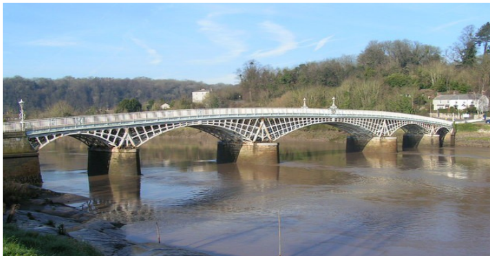
Chepstow Bridge (Rastrick 1816) – 10-20-34-20-10 m
