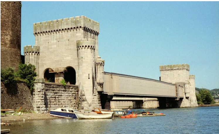
The Conway box bridge (Stephenson 1849) - 141m
