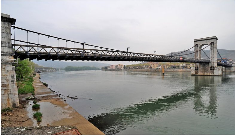
Rhône Bridge at Tournon (Séguin 1825)
