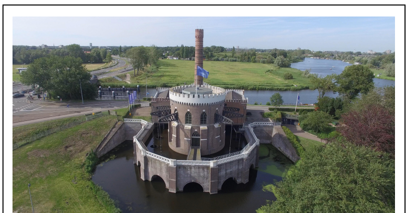
Cruquius pumping station
