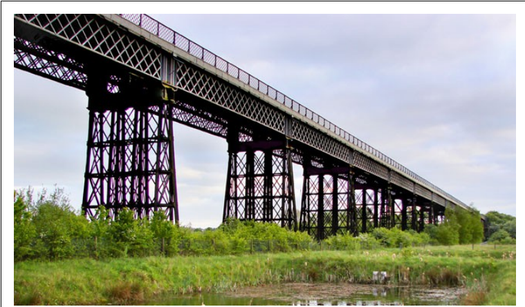
Bennerley Viaduct (1877) – 16 × 23.5 m
