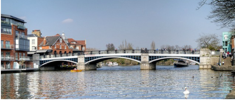
Windsor Bridge (Hollis 1824) – 13-17-13 m
