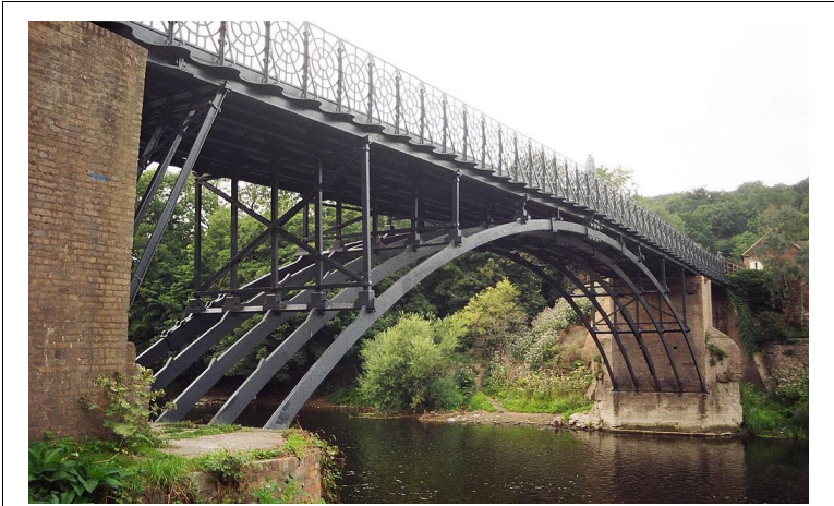
Coalport Bridge (1818) – 32 m
