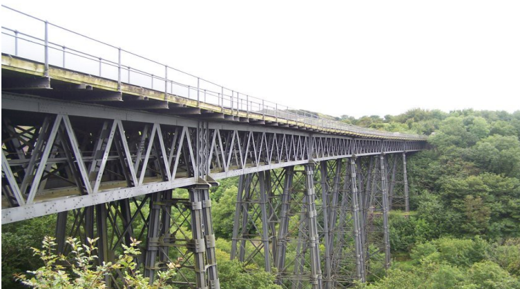
Meldon Viaduct (1874) – 6 × 27 m
