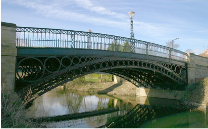
Tickford Bridge (Henry Provis 1810) - 18m
