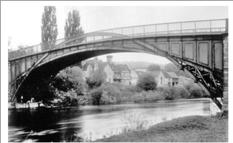
Buildwas bridge (Telford 1796) - 40m
