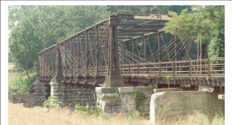
Bollman Truss Railroad Bridge (Unknown 1869)
