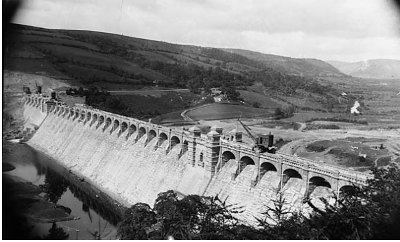
Vyrnwy dam under construction
