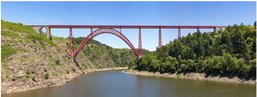
Garabit Viaduct (Eiffel 1885) – 165 m
